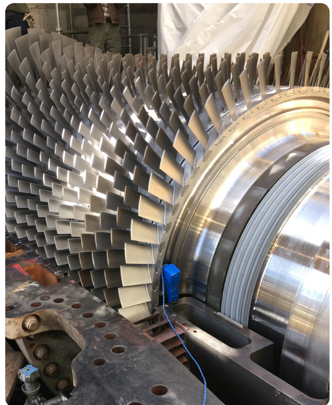
SEED ROTOR INSTALLED AFTER COMPRESSOR
