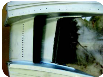
CUTOUT DAMAGED MATERIAL
