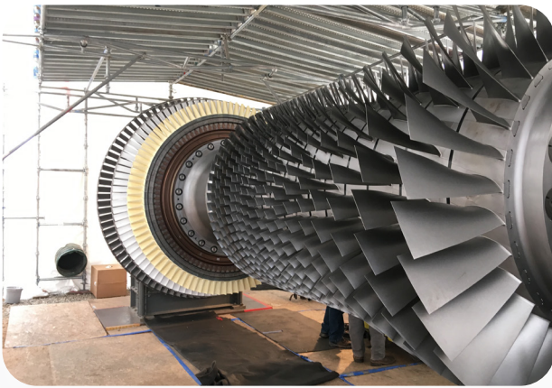
PSM SEED ROTOR INSTALLED WITH NEW ROW 9-17 COMPRESSOR WHEELS
