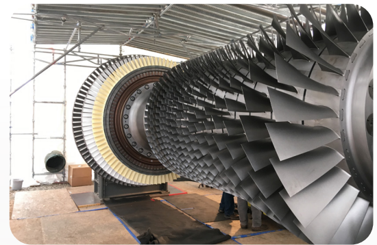
PSM SEED ROTOR INSTALLED WITH NEW ROW 9-17 COMPRESSOR WHEELS
